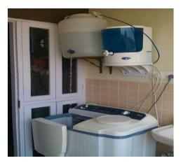
> Water Purifier with Storage tank, which allows the waste water to be reused appropriately. Since while the water is not good for drinking it is perfectly fine for washing clothes.
